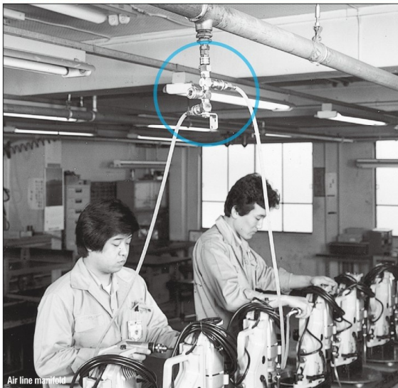
Air line manifold
