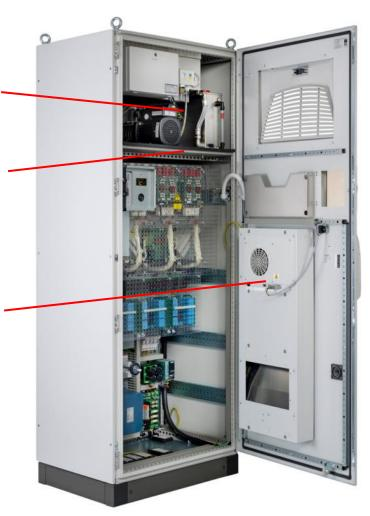
Fig. 3: Cooling equipment (ECOsine® active FN34xx-200/250/300-xxx-x)
