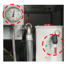
Fig. 6: Pressure and filling level indication of the cooling circuit
