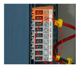
Fig. 8: Terminals for auxiliary power supply
