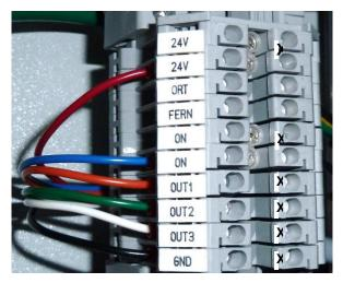
Fig. 64: X5a terminal strip – digital inputs and outputs (ECOsine® active 200/250/300-xxx-x)
